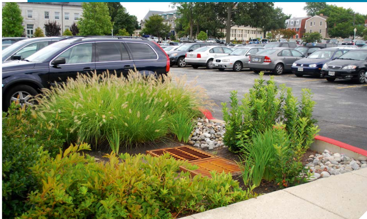
Rain garden in a parking lot.
