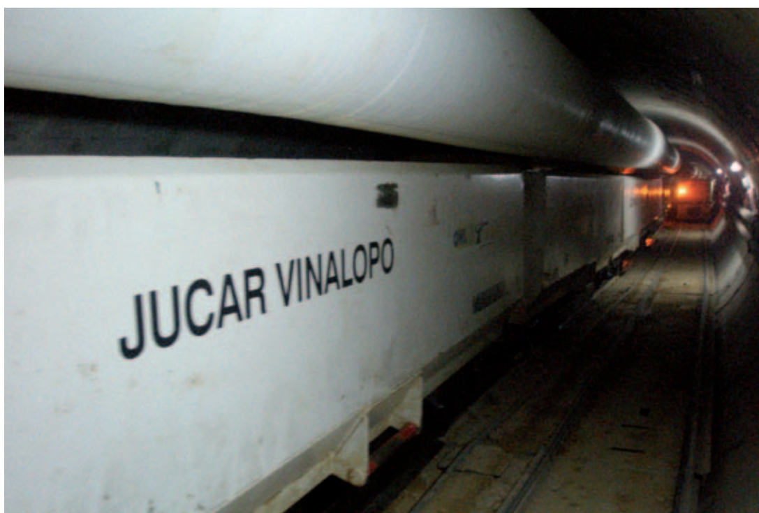
Tunel Corbera. Vagonetas (Tramo B).
