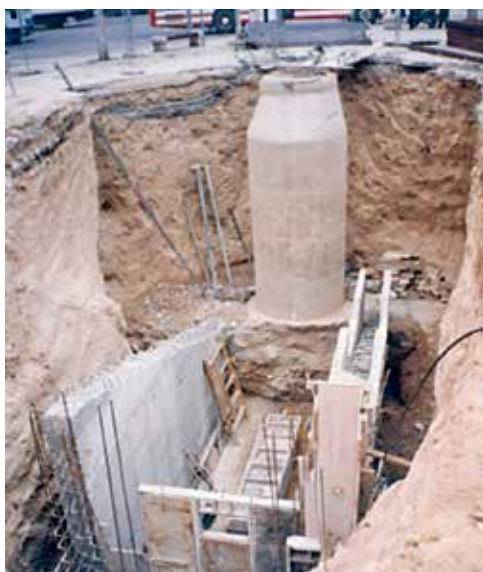
Image 8. Channelling the sewerage network in Calle Fernando Madroñal – Connection with Parque collector
