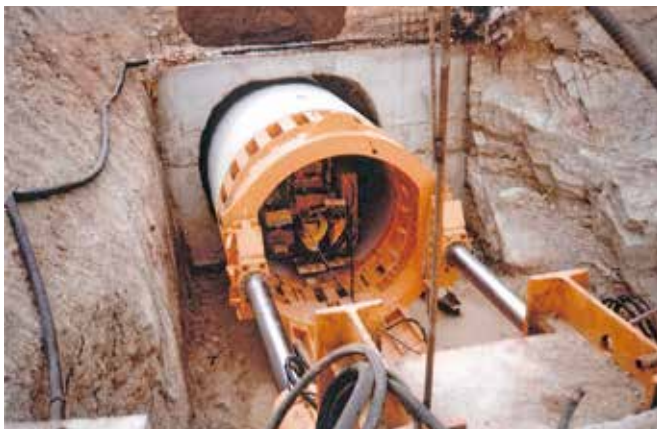
Image 7. Replacing general collector for Section I – Driving Ø2500 under the Gran Vía
