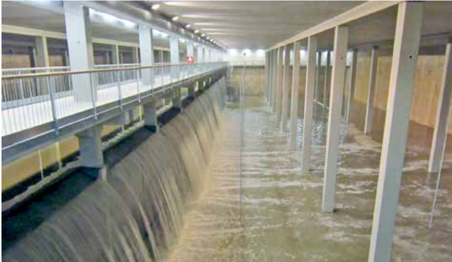
Image 9. The José Manuel Obrero Anti-Pollution Tank operating after a period of heavy rain in the City of Alicante
